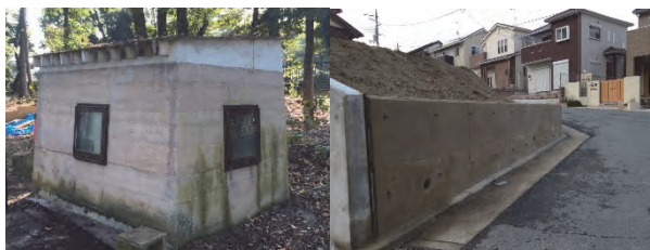
Fig.1 House and retaining wall using PVA fiber.
